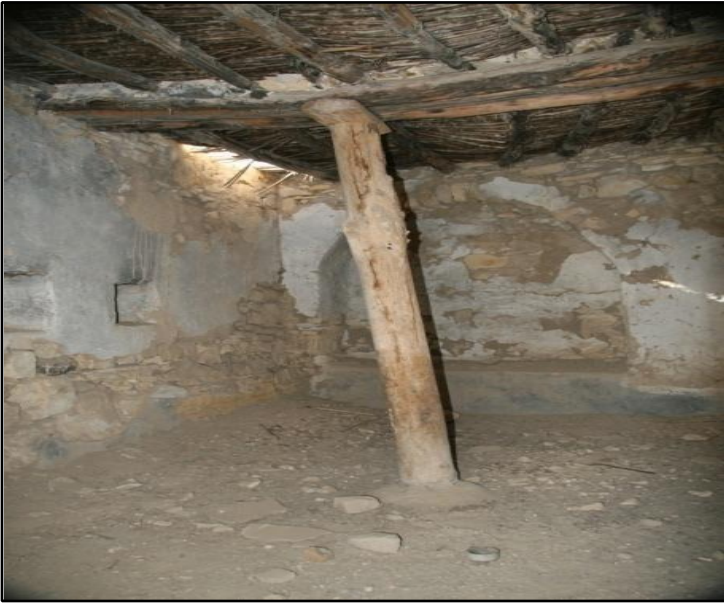
FIGURE 13: Wooden Posts supporting the roofs at Shammakh
