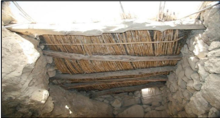
FIGURE 14: Wooden beams and reeds as Roofing materials Shammakh
