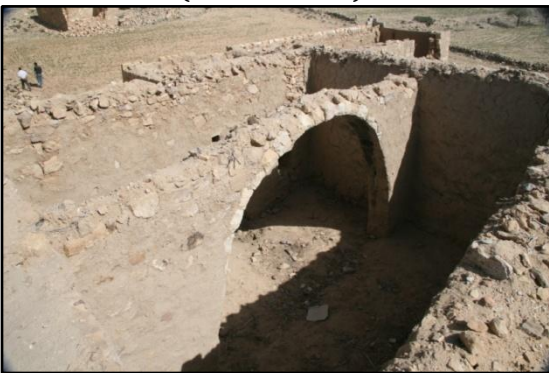
FIGURE 12: Roofing System based on Arches at Shammakh
