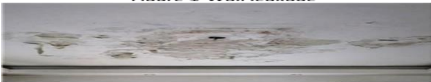
Figure 2: Roof leakage
