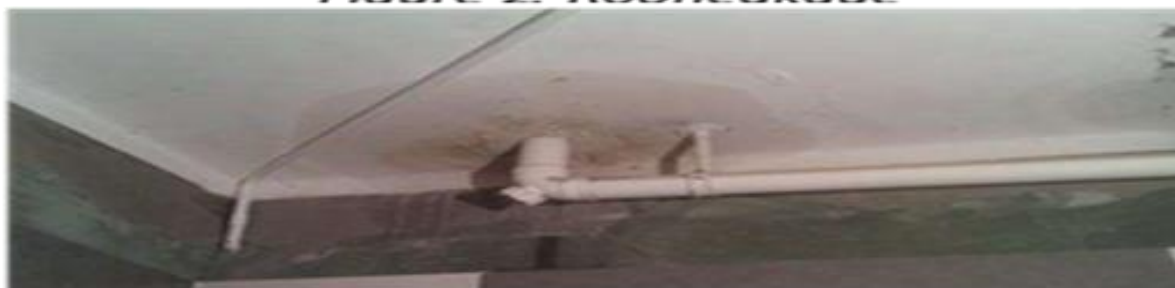
Figure 3: Kitchen and toilet leakage
