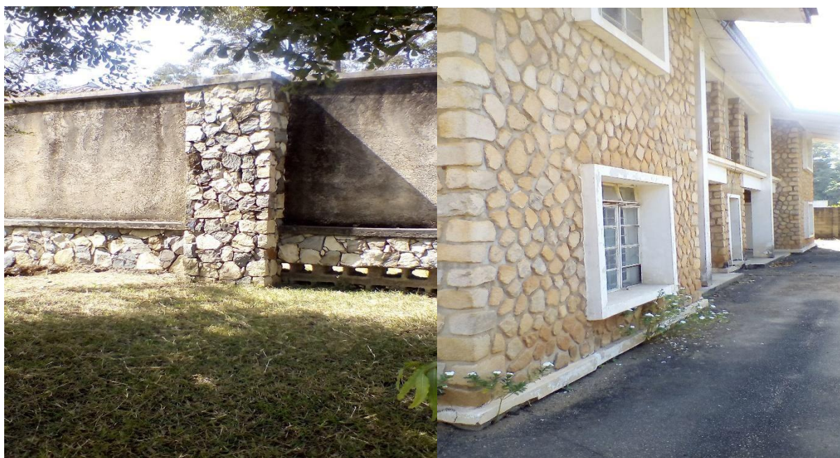
Plate xv: A mortared stone wall made from Limestone used for fencing at G.R.A. Jos.
